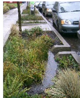
Rain garden between sidewalk and curb; phyto-remediation diagram
